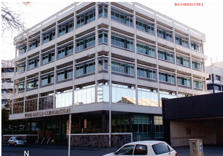
Figure 8-1 Photograph of Pyne Gould Corporation Building prior to collapse (from Jury and Sharpe, 2011, North arrow added).
