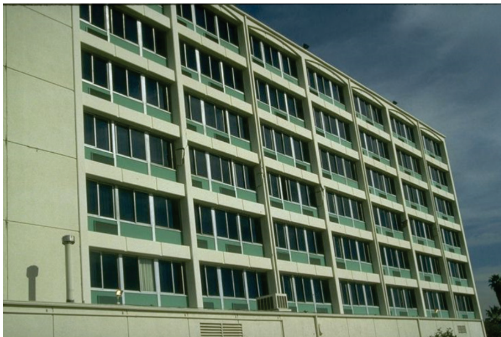
Figure 7-1 Photograph of reinforced concrete moment frame building in Van Nuys.
