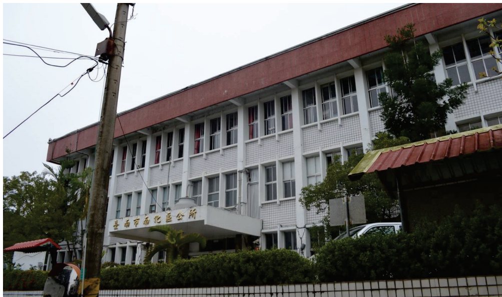
Figure 9-1 Photograph of building from the south (Pujol et al. 2017).
