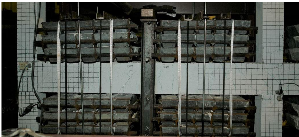
Figure 3-19 Column D1 (left) and column C1 (right) observations after Dynamic Test 1 at Level 1.
