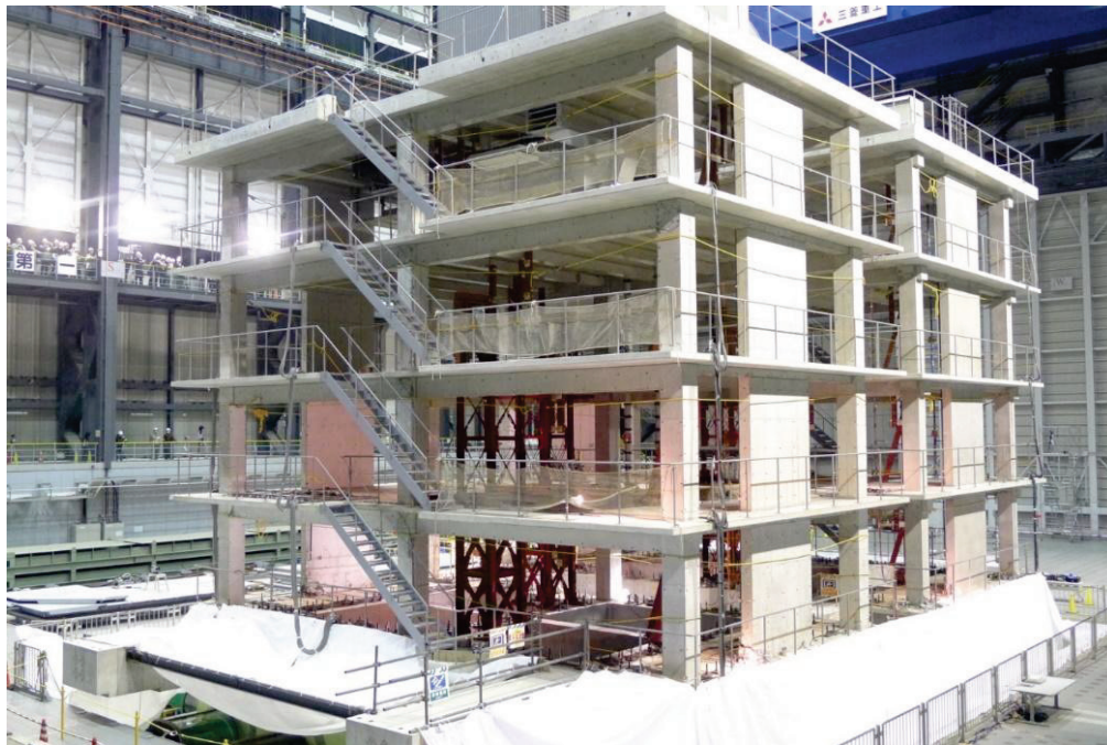
Figure 4-1 Two structures tested at E-Defense shake table, study structure is on the left side of the photo. (Nagae et al., 2015).
