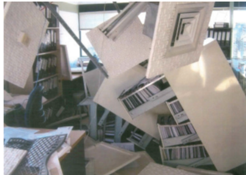
(a) Nonstructural damage
