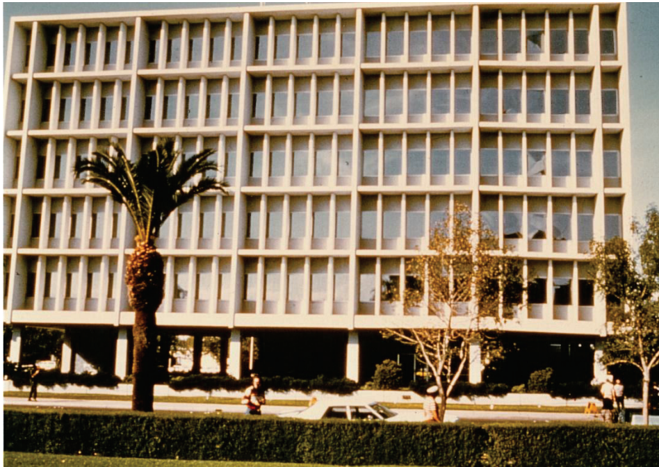
Figure 6-1 Photograph of Imperial County Services Building in Imperial County, California (ATC, 1984).
